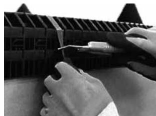
1. First of all grasp the foil and cut it open with a cutter knife. Make sure the blade does not make contact with any of the panels to not damage them.
