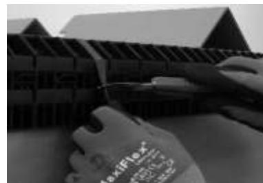
1. First of all grasp the foil and cut it open with a cutter knife. Make sure the blade does not make contact with any of the panels to not damage them.
